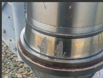
High speed shaft bearing damage detected using ecoCMS
