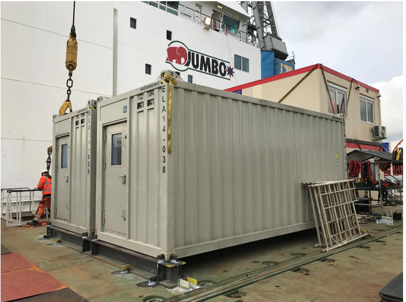
The ELA Offshore Living Quarters were installed on board MV Fairplayer.
