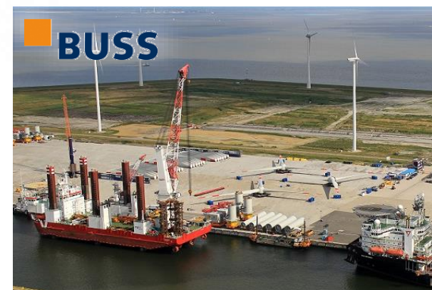
2020: Buss Terminal Eemshaven provides Marshalling Port Services for Foundations of Hornsea II (UK)
